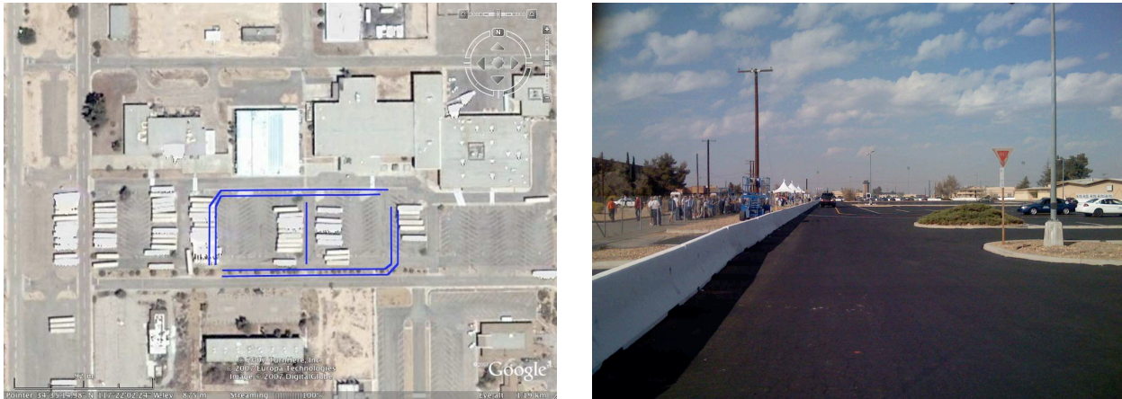
Figure 14: Test Area A
