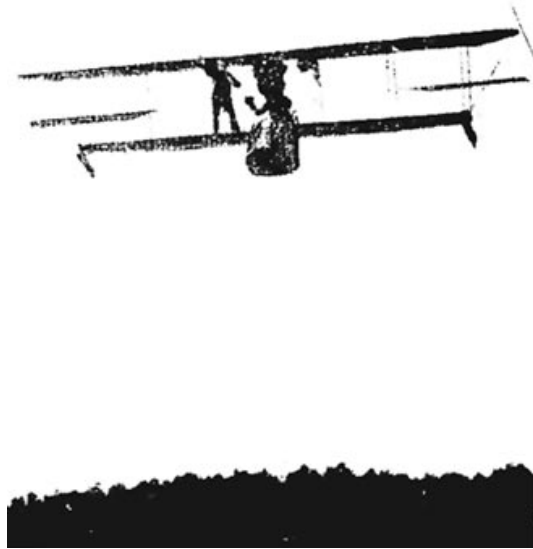
Figure 1.11 Picture from Sperry's contest in Paris. Sperry's son is at the stick and the mechanic walks on the wings to introduce disturbances. Notice the proximity to the ground.
